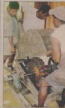
INSTALLATION: Islanders do the hard work on installing a hydro-turbine.
