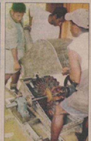
INSTALLATION: Islanders do the hard work on installing a hydro-turbine.
