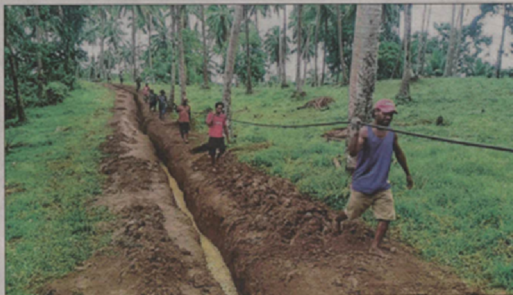
Local helpers carrying HV cable from the village of Tam to step up
